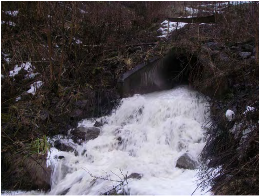
Photograph 1: Burlington International Airport (March 11, 2009 sample), Station D018.
