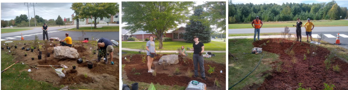
Fig 3: Community volunteers, Milton municipal staff and WNRCD communications intern help to install perennial plants in a new rain garden at the Milton Municipal Building.
