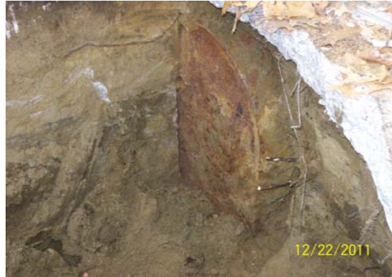
Plate 2 Eastern side of UST exposed
