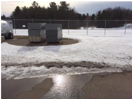
Photograph F-5. Valley West Apron (Facing southwest)
