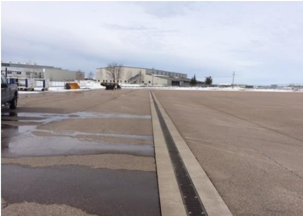
Photograph 3-2. View of southwestern side of Apron
