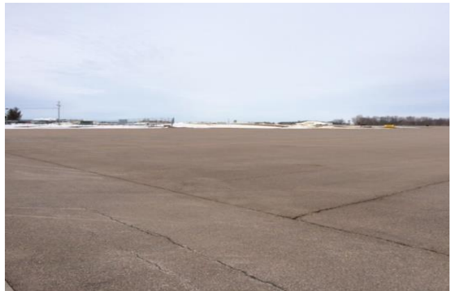
Photograph 3-3. View of the Apron looking northeast
