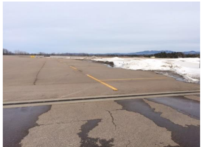
Photograph 3-1. View of the Apron looking east
