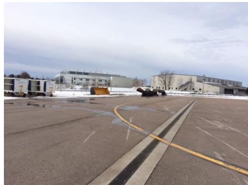
Photograph F-4. Valley West Apron (Facing southwest of Apron)
